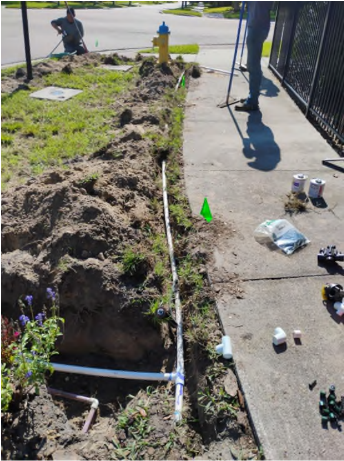
New irrigation installation at entrance to West Lake
