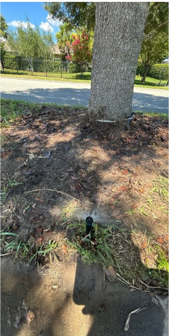
M36 completed repair
